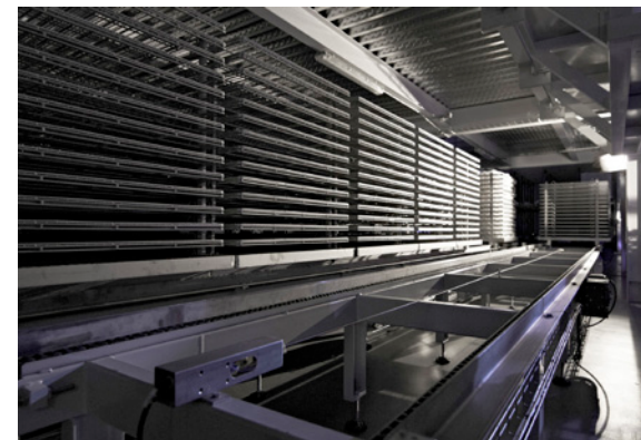
Parenteral solutions production plant. Murcia, Spain
