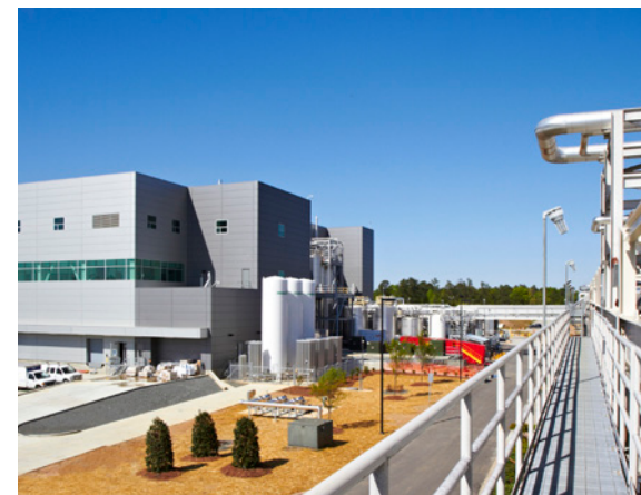
New fractionation plant. Clayton, NC, USA
